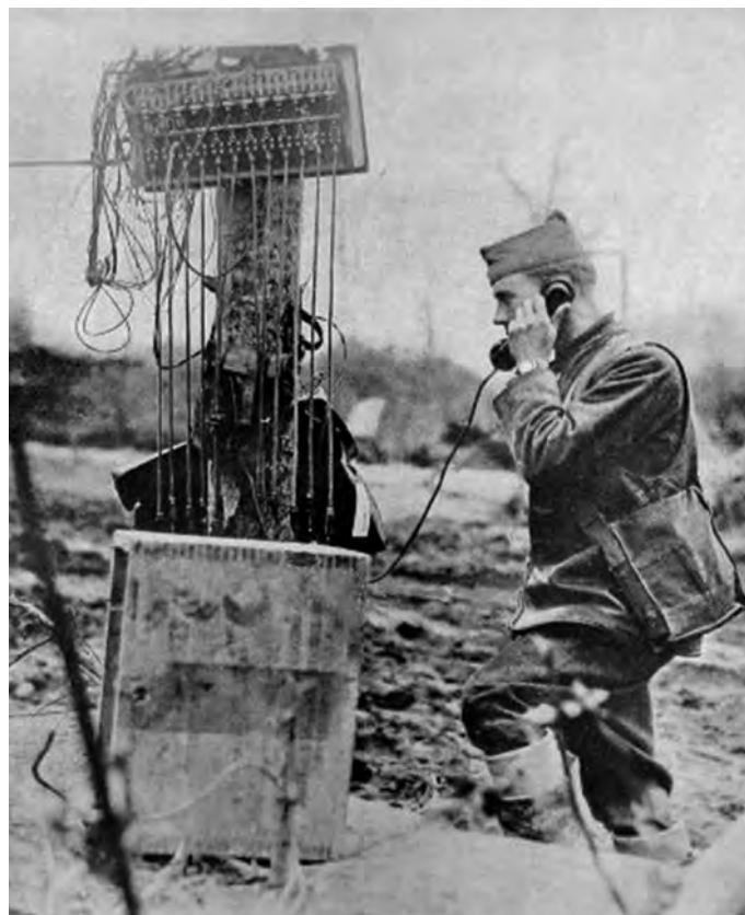
US Field Telephone Exchange
