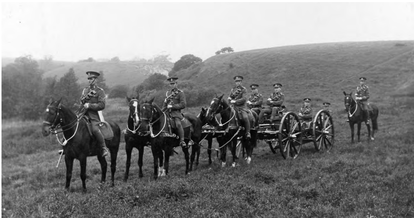
The Cable Wagon was first used to lay cable in the Crimean war. Before the battle of the Somme over 50,000 miles of cable were laid, 43,000 miles above the ground and 7,000 miles of armoured cable dug in to a depth of six feet.
