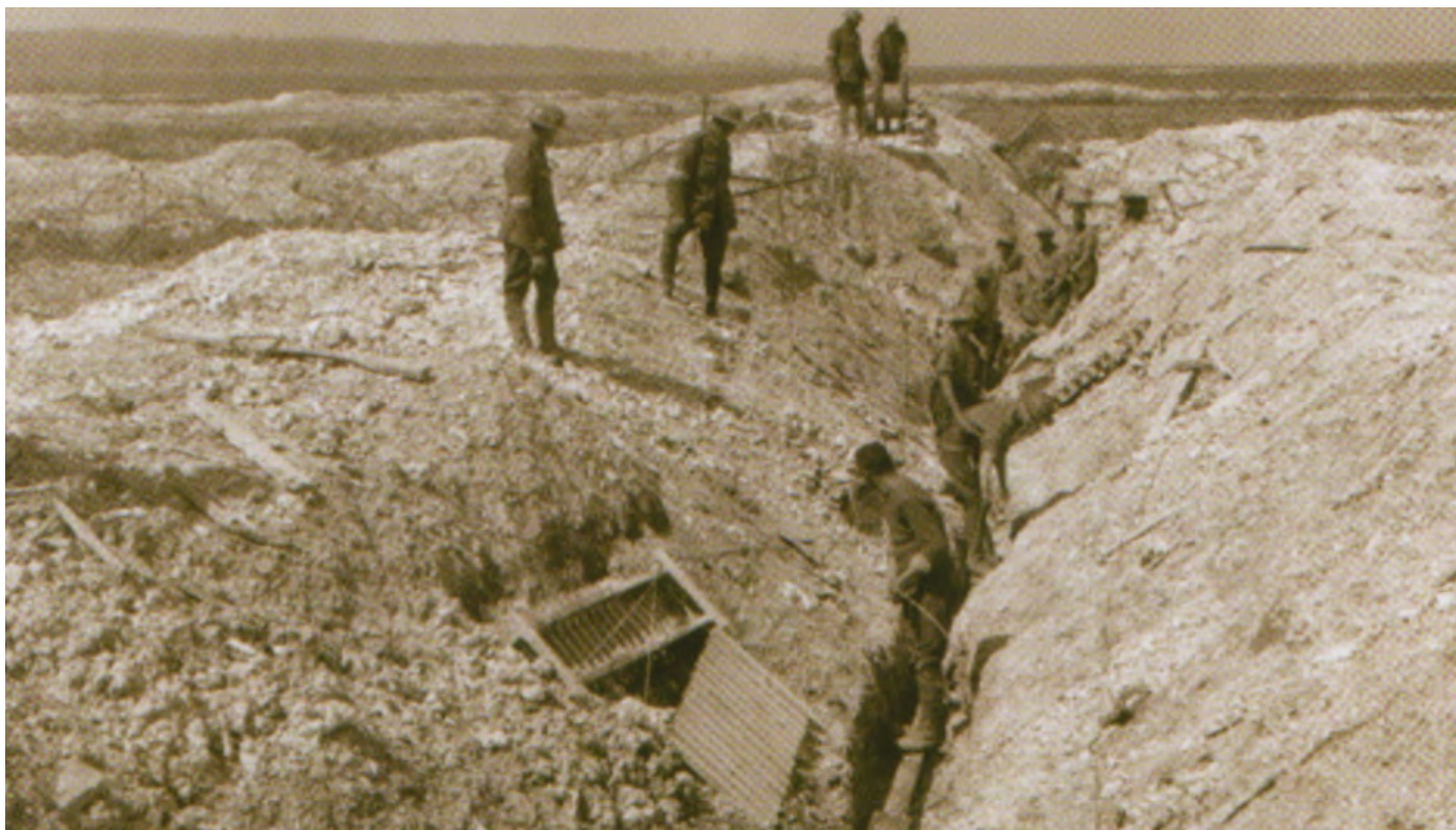
Laying armoured cable
